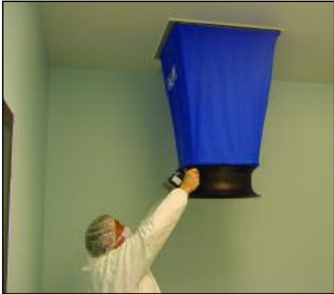
Hood being used to measure air volume coming from an air supply diffuser
